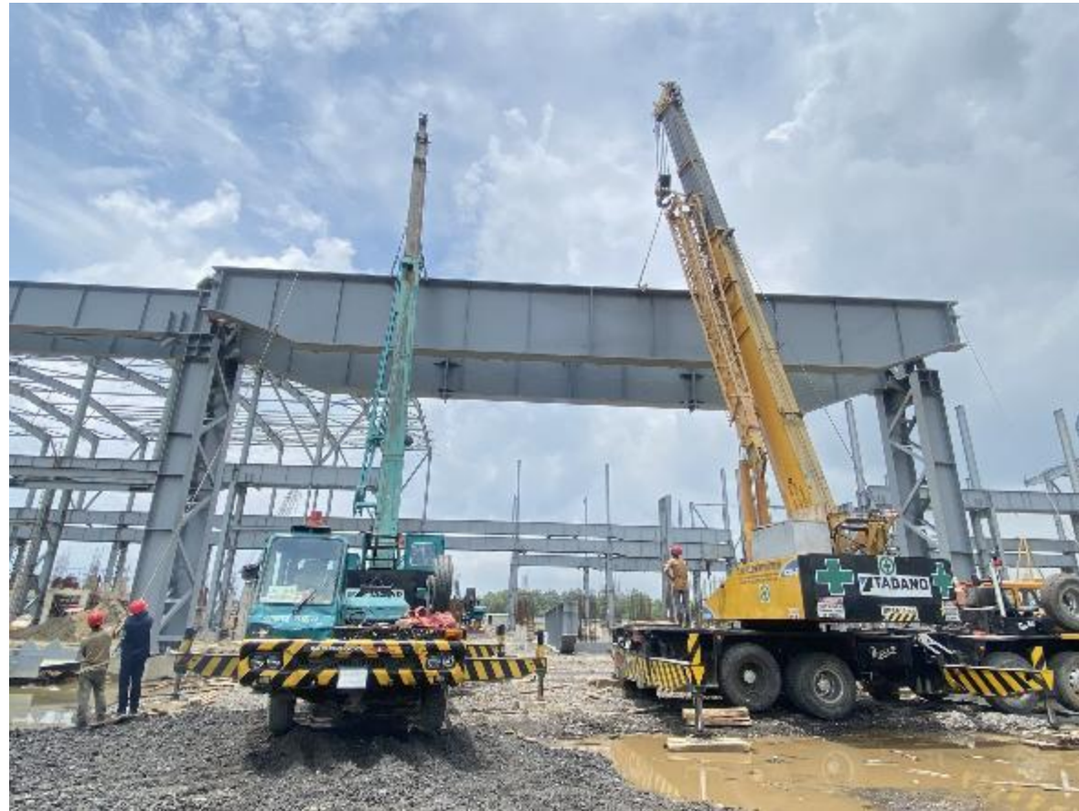
24m crane beam under fabrication
