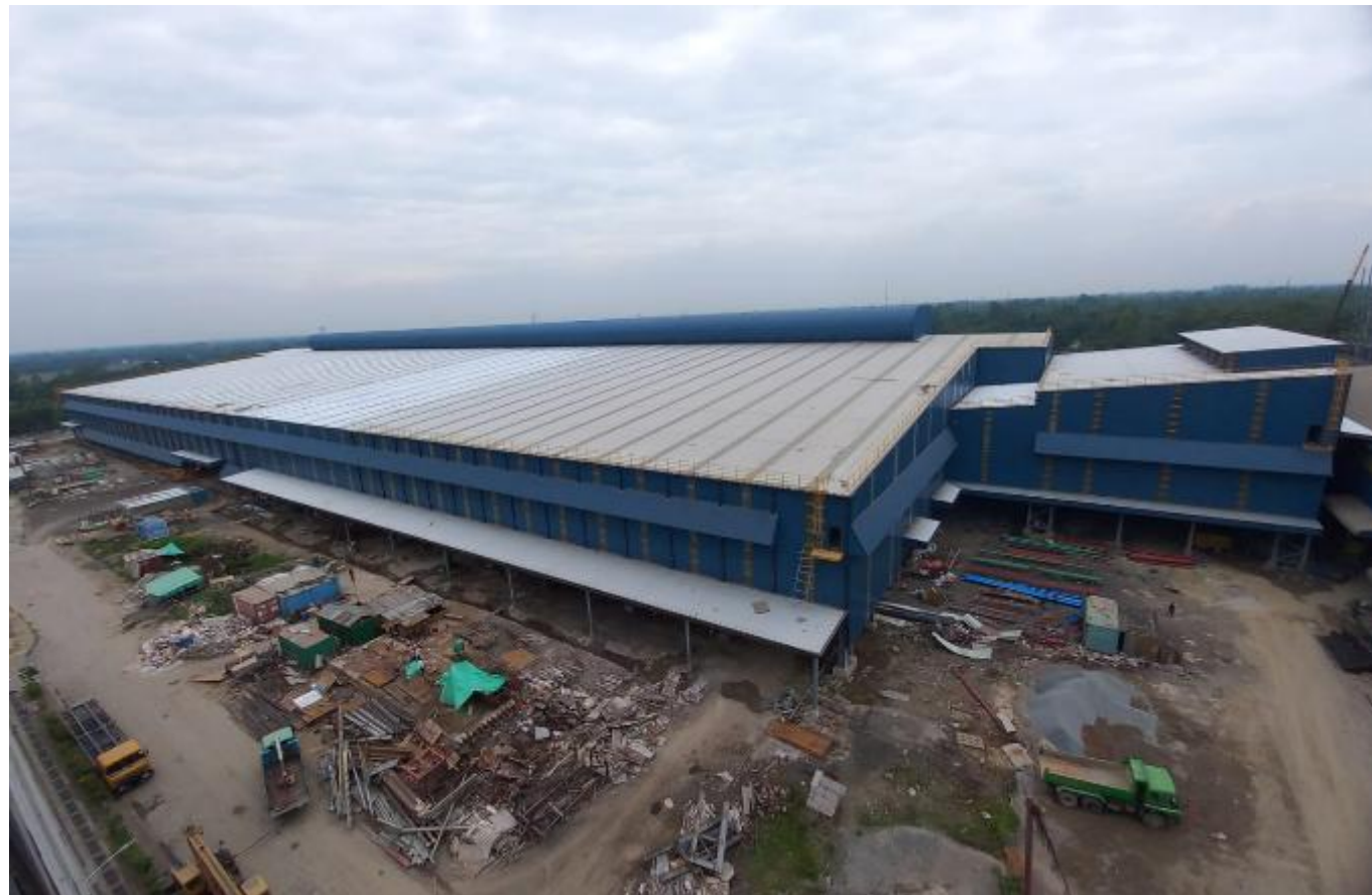
BSRM Steel Re Rolling Mills (Phase 3)
