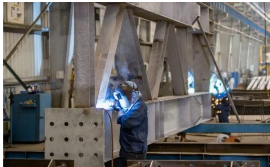
07.B Finishing Product – Lacing Column Final welding and inspection for lacing column
