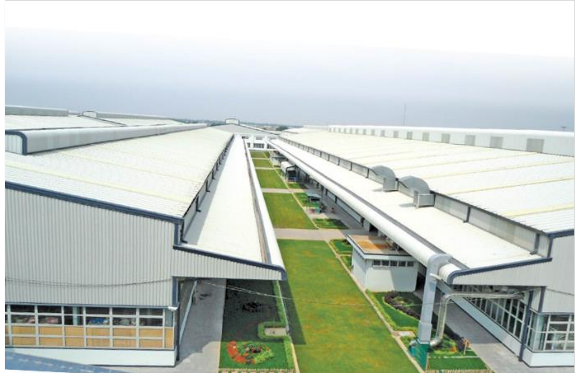
Taekwang Vina Moc Bai, Vietnam Shoes factory achieved LEED Silver for Green Building
