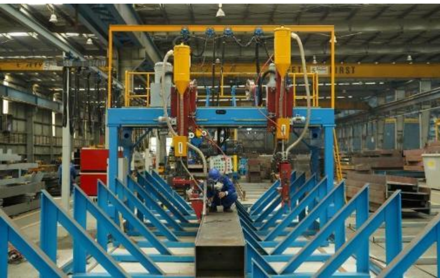
03-C Box Welding For assembling closed-section beams with high strength and stability
